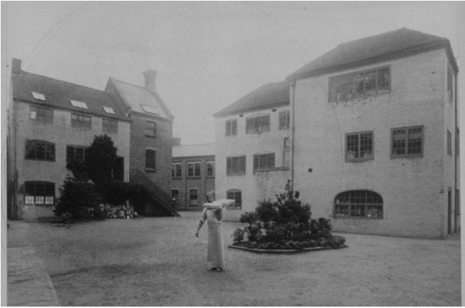
Some of Chamberlains buildings before demolition in the early 1930s
